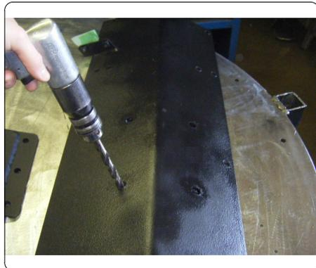
5. Trim foam on skid plate to allow clearance for 1/2" flange nuts at (4) mounting locations.
