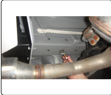
4. Raise hitch into position and pull the fishwires and carriage bolts through the side plates. **Note:** Feed the fishwires through the mouting holes while raising the hitch. Remove the fishwires from the carriage bolts and secure the hitch with 7/16" flange nuts.
